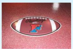
The graphic is embedded in the epoxy coating and protected with a durable, transparent top coat.
